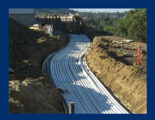
In this first installment of WS's new series exploring the "fine points" of watershape construction, Kevin Cobabe gets down to basics about running multiple pipes in trenches. As simple as it seems, he says, there are a handful of key issues that are important to keep top of mind when working beneath your feet.
