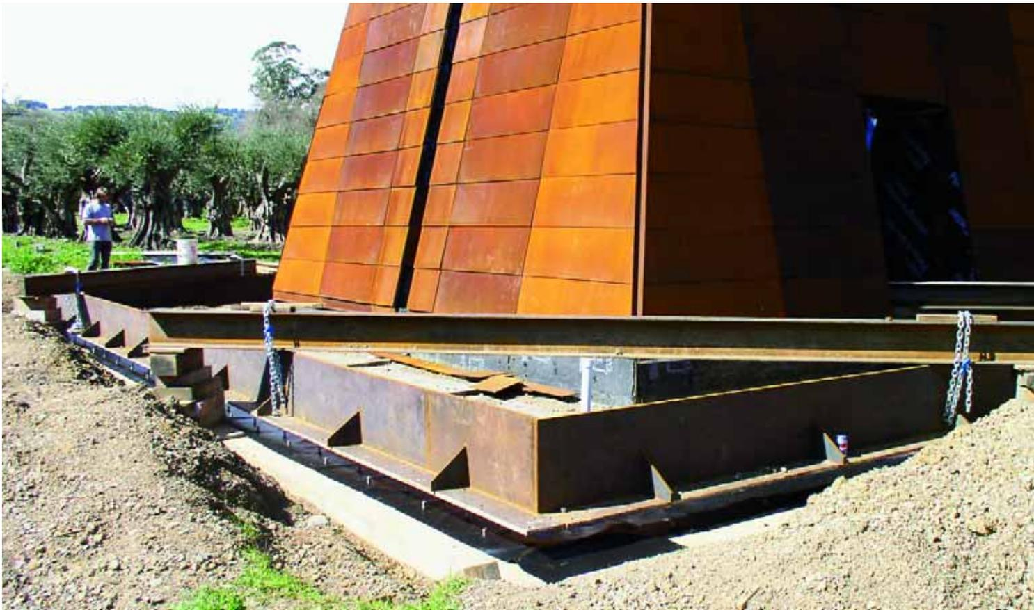
steel. (Cor-Ten is a carbon steel that rusts just on the surface: The thin layer of rust protects the underlying steel from rusting as well.) The house features a cantilevered roof corner that called for use of #18 rebar (with a diameter of 2-1/8 inches) to support it. Around the home, the landscape architect had distributed 36 specimen olive trees that had been moved onto the site.
