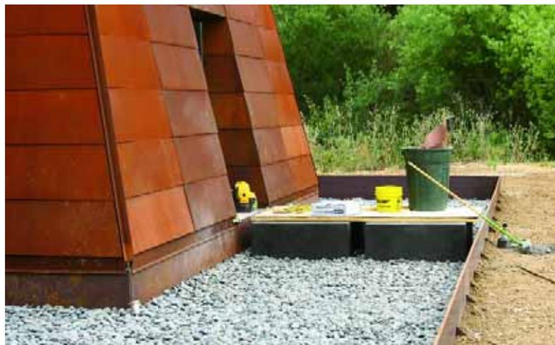
Once the liner was fully in place, we filled the basin with smooth stones and then water-tested the system. After we dealt with a few leaks that developed in the installation process, the system was ready to go.
