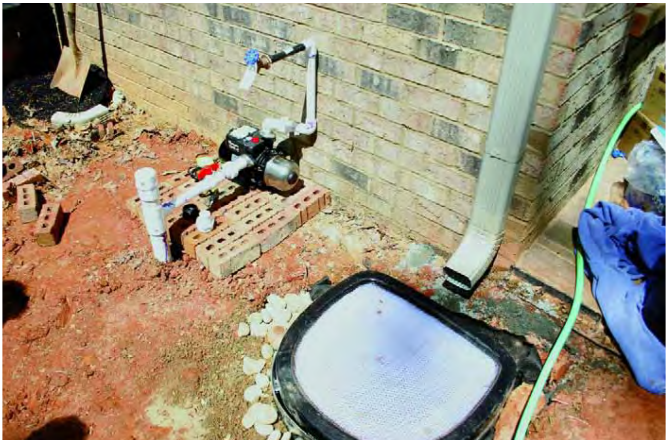
Lots of the rainwater falling on the landscape has the opportunity to find its way into the harvesting loop, but the largest direct contribution to the reservoir comes from rain that falls on the home's roof and flows to its downspouts. To capture that water at the bottom of the system, we set up a pre-filtering unit that allows water to flow directly to the reservoir. Seen to the left of the completed installation is a booster pump that feeds water to a hose bib and allows the homeowners to use some of their stored water for irrigation.
