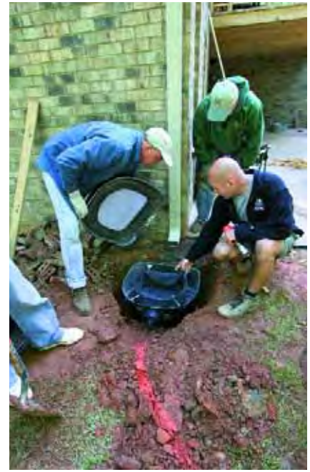
Lots of the rainwater falling on the landscape has the opportunity to find its way into the harvesting loop, but the largest direct contribution to the reservoir comes from rain that falls on the home's roof and flows to its downspouts. To capture that water at the bottom of the system, we set up a pre-filtering unit that allows water to flow directly to the reservoir. Seen to the left of the completed installation is a booster pump that feeds water to a hose bib and allows the homeowners to use some of their stored water for irrigation.
