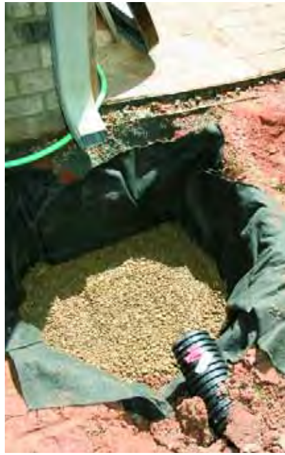
Lots of the rainwater falling on the landscape has the opportunity to find its way into the harvesting loop, but the largest direct contribution to the reservoir comes from rain that falls on the home's roof and flows to its downspouts. To capture that water at the bottom of the system, we set up a pre-filtering unit that allows water to flow directly to the reservoir. Seen to the left of the completed installation is a booster pump that feeds water to a hose bib and allows the homeowners to use some of their stored water for irrigation.
