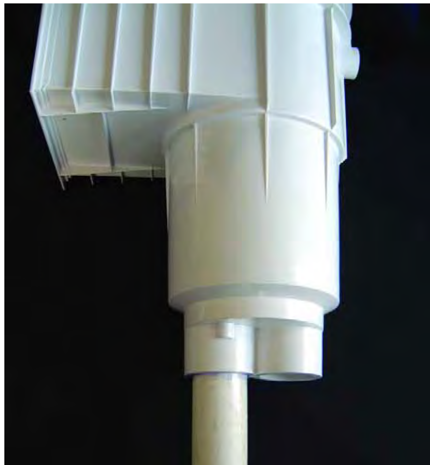
Figure 5: Connections between dissimilar materials are most often found where pipes tie into equipment or as shown here, where PVC piping is connected to an ABS skimmer.
