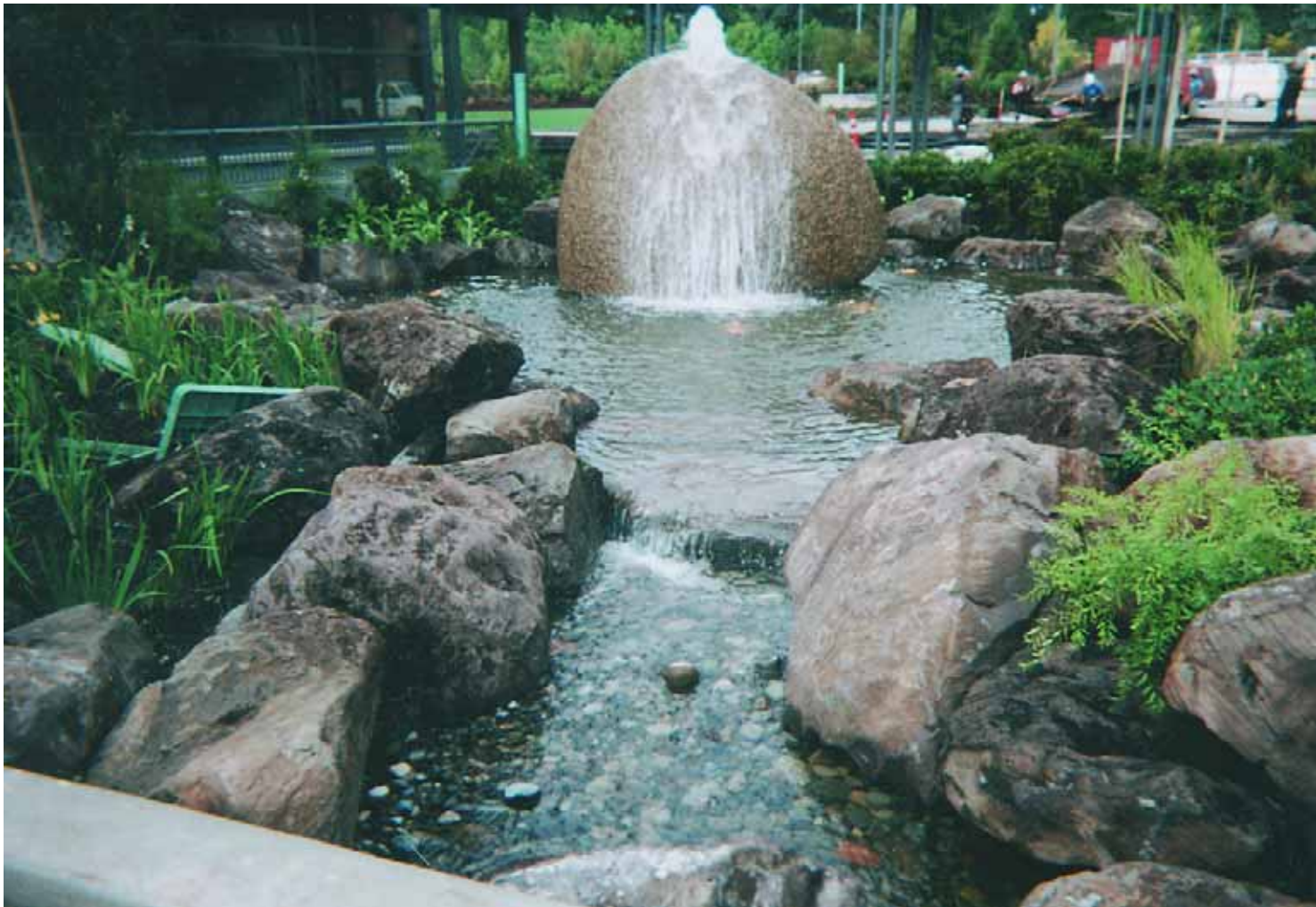
The Mother Stone would appear to be the source of all the water that flows through the system, but that's far from the case: Just 50 gpm flow up and through the stone in a system that has a total flow of 4,500 gpm.
