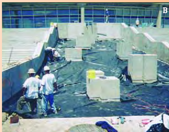
PRELIMINARIES: By the time we arrived on site, the general contractor had set up a platform for our work as well as the support structures for the seven bronco sculptures (A). We came in and put down
