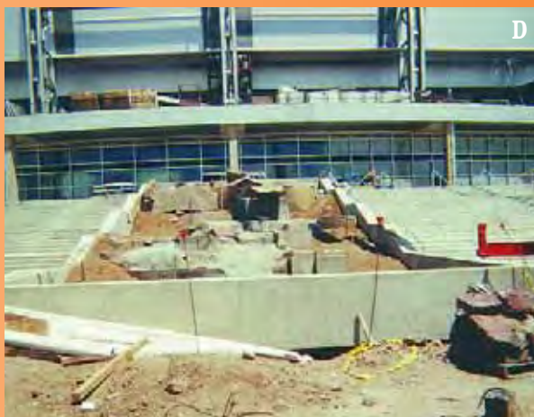
a liner to protect the adjacent stairways from any possible undermining (B), then added soil to create rough contours (C) before setting up the shotcrete shell (D) and moving in the boulders (E).
