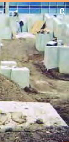
a liner to protect the adjacent stairways from any possible undermining (B), then added soil to create rough contours (C) before setting up the shotcrete shell (D) and moving in the boulders (E).
