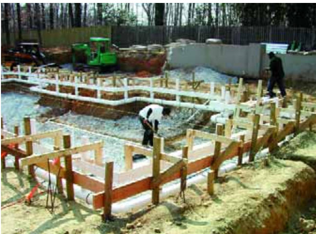
In combination with the pool's long perimeter, the repeated 90-degree turns in the edge detailing made for unusual challenges in designing and installing the trunk lines for the gravity-fed overflow system. In all, four separate lines feed the surge tank.
