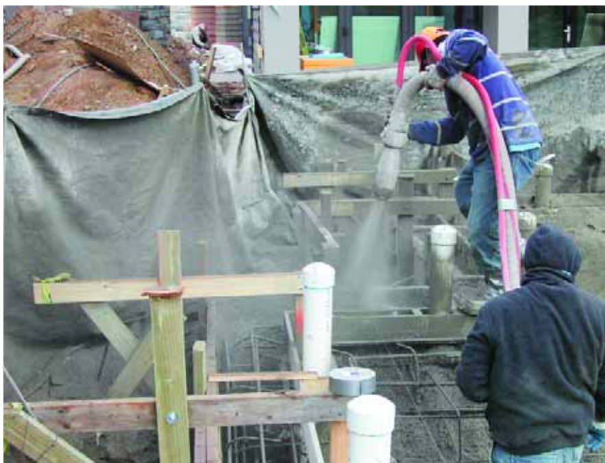
Shooting the shell was another challenging process, simply because there was so much going on in the walls of the pool and the bond beam. When the process was complete, we removed the gutter forms and armature and began working on the finish details.
