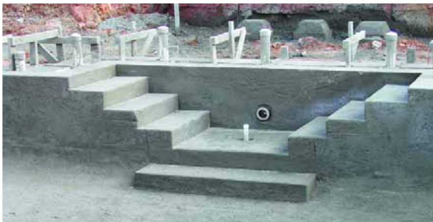
Shooting the shell was another challenging process, simply because there was so much going on in the walls of the pool and the bond beam. When the process was complete, we removed the gutter forms and armature and began working on the finish details.
