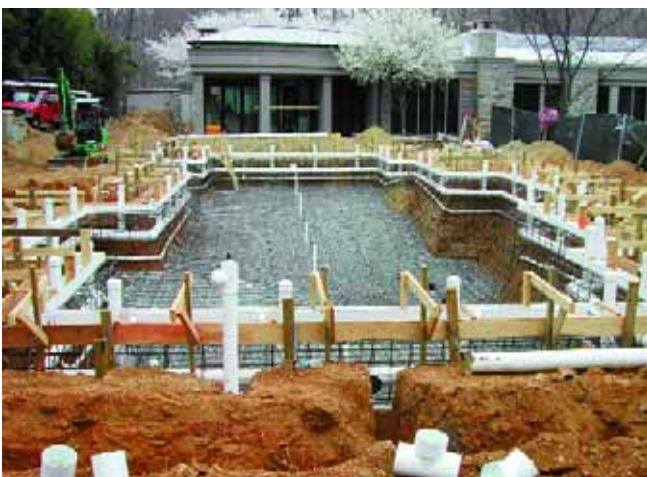
In combination with the pool's long perimeter, the repeated 90-degree turns in the edge detailing made for unusual challenges in designing and installing the trunk lines for the gravity-fed overflow system. In all, four separate lines feed the surge tank.
