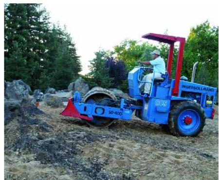
We started on site with a literal blank slate – a flat, featureless lot. But the trees on an adjoining property helped us set the pattern for a massive contouring process that ultimately saw us bring in 16,000 tons of soil, every grain of which we carefully compacted into place.
