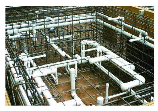
At this point, everything is ready to go: spacers and dobies are all in place, the steel has been tied to the forms, the plumbing has been secured and we've done all we can to make certain that the concrete-application process will move forward with negligible vibration and we can be assured the steel will be completely encapsulated.
