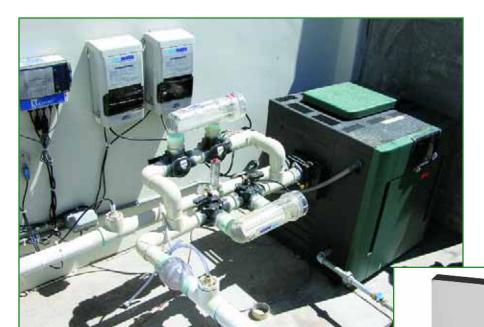
The improper installation of one of these salt-chlorination cells is what led us to get involved in detailing our equipment sets in three dimensions. (Notice that one cell is installed in the correct upright position and that the other is at about a 90-degree angle, despite the supplier's recommendation.) Working in three dimensions, we were able, without taking up any additional space, to illustrate a better way to get the job done and allow both cells to produce the same level of chlorine.
