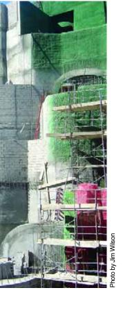
structure – some of them up to 20 feet deep – we used a liquid waterproofing material that was rolled on and also set up a high-performance drainage system that uses Flat Pipe, a technology we've developed for these sorts of applications.
