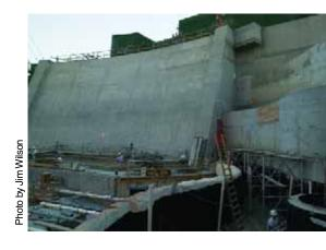
The giant waterwall and its pond are central fixtures on the hotel grounds. They had to be waterproofed, of course, and so did the planters that flank the waterwall on numerous levels – each pocket requiring extensive waterproofing with asphalt-based membranes.
